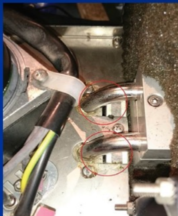
Holes by the flow and return pipes
